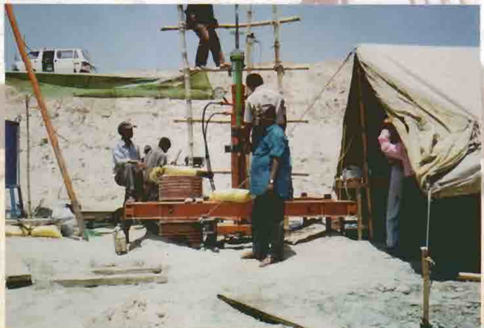
Electric Cone Penetration Test for Paksey Bridge Construction Project.
