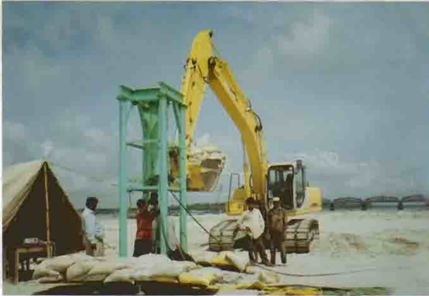
Electric Cone Penetration Test for Paksey Bridge Construction Project.
