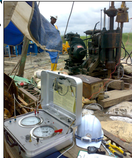
Offshore Electronic CPT Testing
